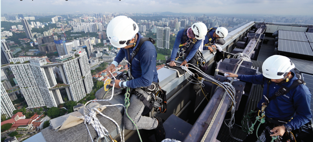
A team of five cleaners from facade restoration firm Renuglass perform cleaning works at Guoco Tower by hand
