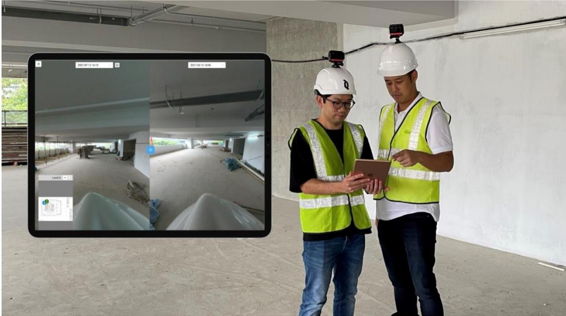
*Figure 4: Airsquire's AirGo platform enables project managers to check and compare 360-degree site progress inspection photos of projects under construction and share them with the project team.*
